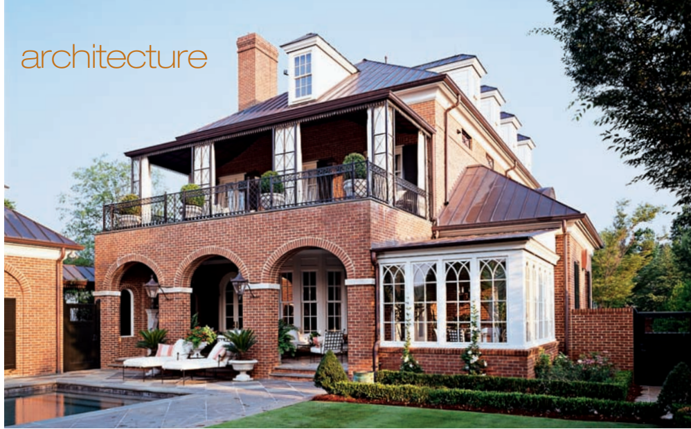
ABOVE: The house widens at the rear to accommodate the kitchen and the adjacent conservatory, which the owners use for casual dining. On the porch off the master bedroom, the latticelike metalwork imitates a Regency signature. A Greek key pattern tops the railing's attenuated ovals.
